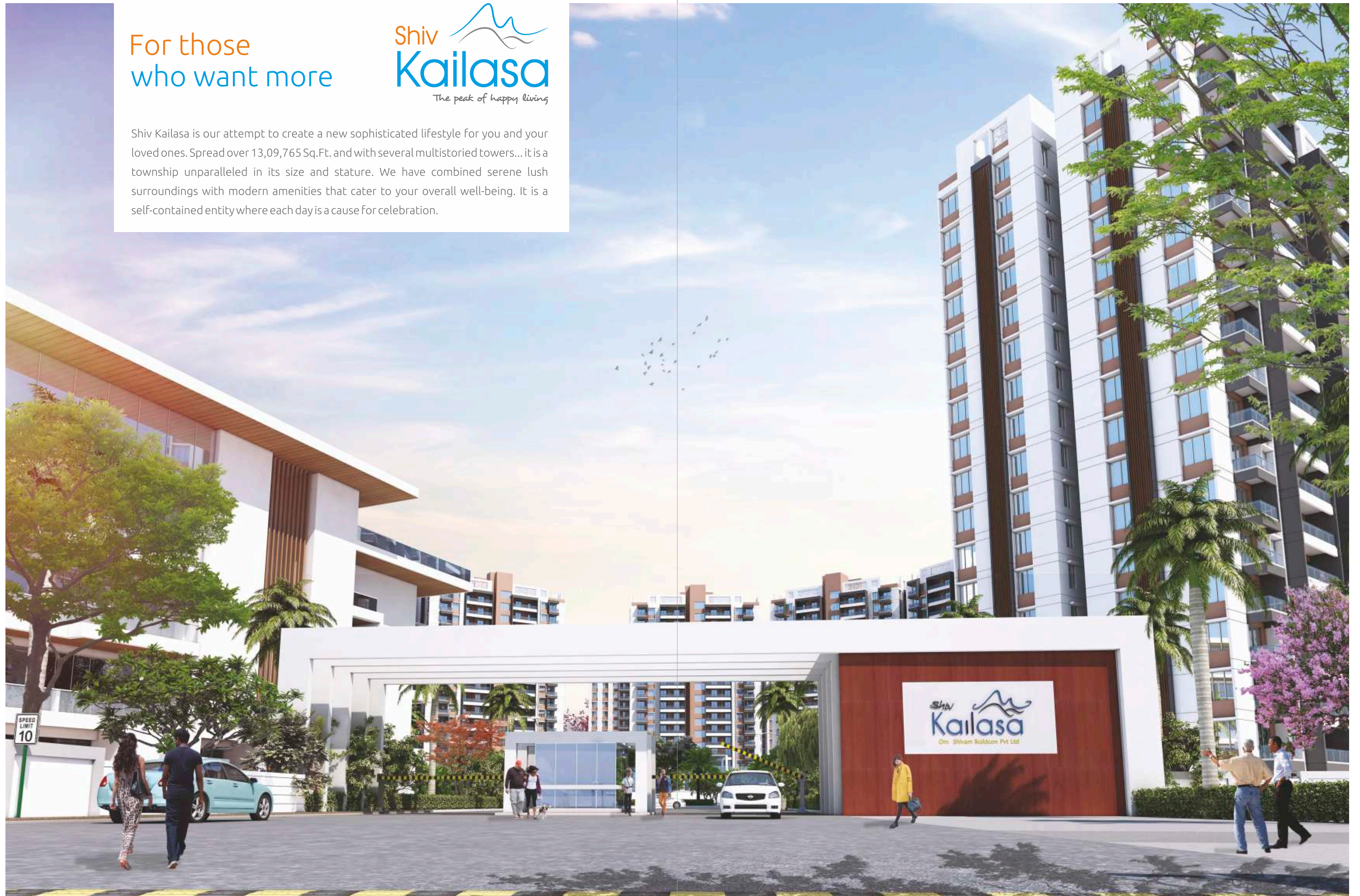
THE GRAND ENTRANCE GATE AND SECURITY CHECK POST WITH BOOM BARRIERS MECHANISM AT SHIV KAILASA
